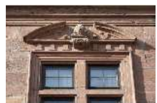
Asch.I, Fensterdetail, DI030290, BSV
