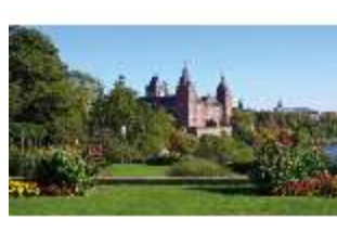
Asch.I, Westfassade, DI011068, BSV
